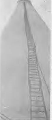
STRETCHING UP , up and up is the 309-foot length of the No. 2 Powerhouse stack; the center picture is a McHugh's-eye view of the ground from those dizzying heights. That's John McHugh at right. The ladder, even though film is in appearance, is amply strong.
